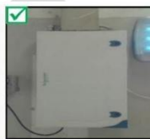
Electrical panel and board should be covered
