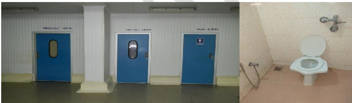
Gender Specific Toilets
